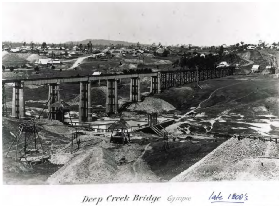
Figure 4.1: Deep Creek Bridge, Gympie (QLD, Australia), showing mining activities within and adjacent to the creek, circa 1890. This bridge is located within 200 m of the Mary River. Photo: State Library Queensland.
