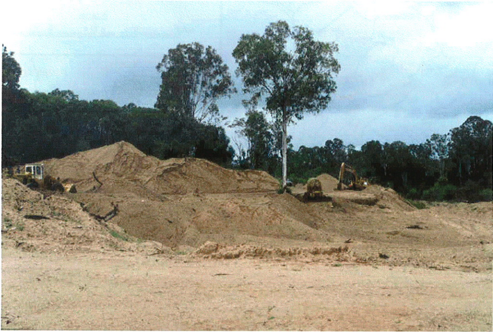
Plate 2.1: Sand and gravel extraction, Tiaro 1998.
